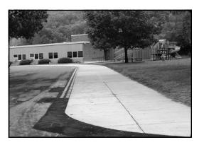
The sidewalk snowmelt system (pictured left) was completed. This system uses the water from the Main Street building boiler to keep the bus loop sidewalk clear of snow and ice. This system saves the District thousands of
